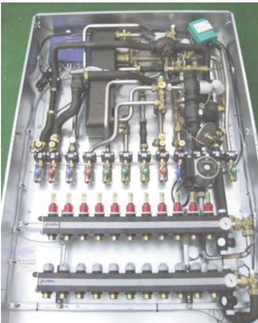
Comfort HIU allows heating or/and cooling + addition heating circuit while summer operation i.e. for bathroom towel heater
